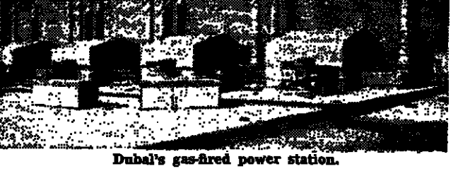
Dubai's gas-fired power station.
